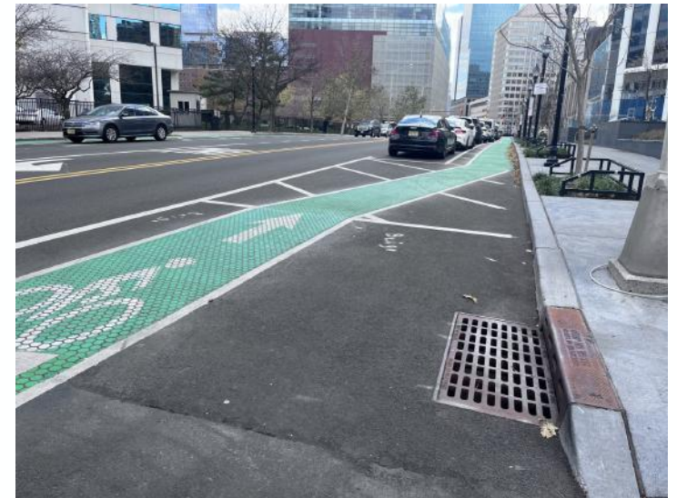
fresh bike lane in downtown Jersey City. Cycling rates have grown as the city has added protected infrastructure. Photo: John Surico/Bloomberg CityLab
